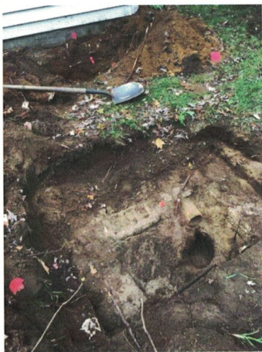
These two photos show the old 1946 septic system that was dug up pending installation of the new septic system.
