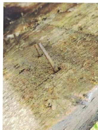
The roofers found square nails in the roof
