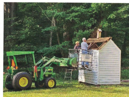
Stripping off rotten roof boards
