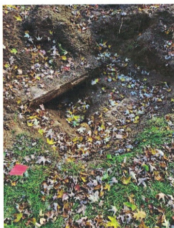
These two photos show the old 1946 septic system that was dug up pending installation of the new septic system.
