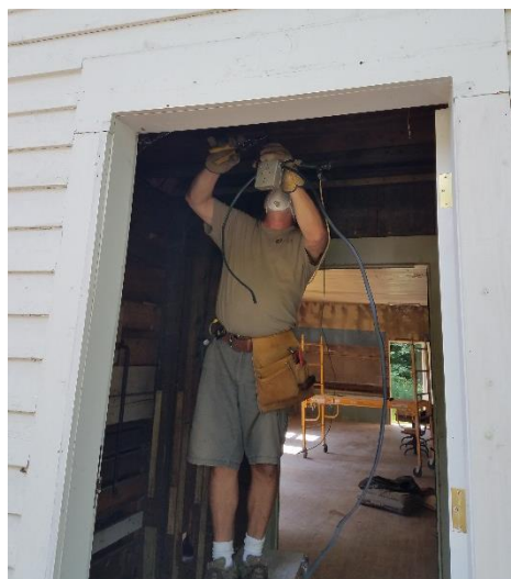
Jim Key tears out old insulation and ceiling and wall boards in the entryway.
