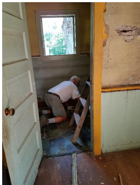
Jim Fitzpatrick removes old wall covering that was mildewed and damaged. He also replaced insulation in the ceiling.
